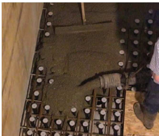
Placement of concrete see page 5 for finished floor.
