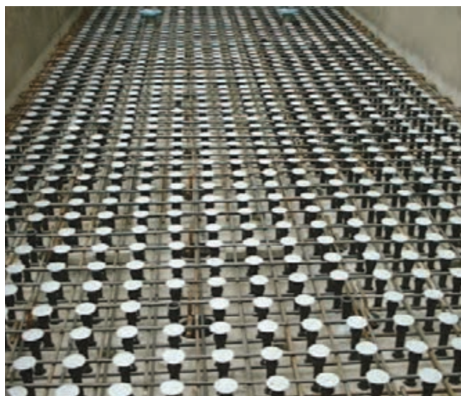
Installed threaded sleeves and protection caps.
