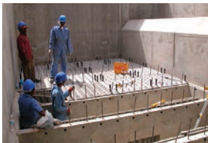
GRC panels being positioned on dwarf walls.
