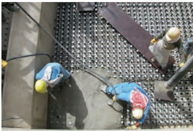
Pouring and vibration of concrete.
