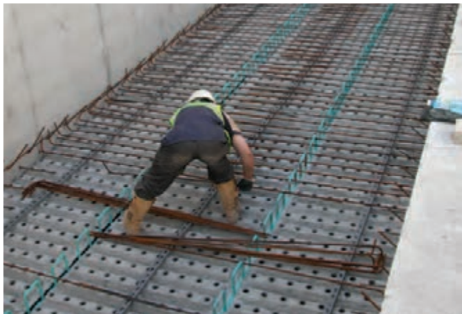
Panels sealed to support wall and abutting panel, then steel reinforcement positioned.
