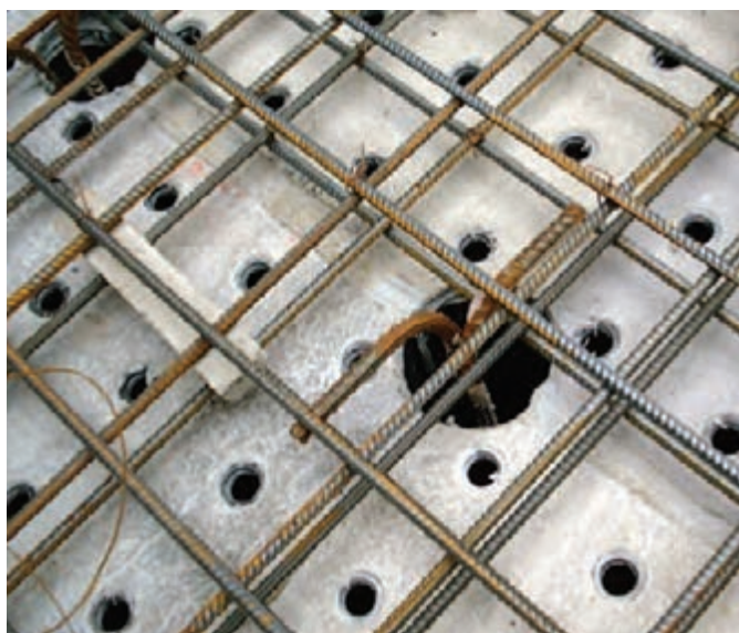
Steel reinforcement showing connecting steel within support tube.
