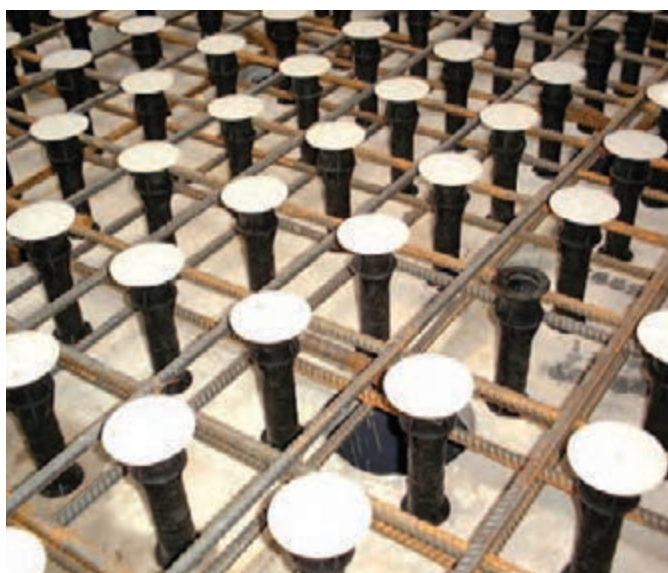
Close up on threaded sleeves and steel reinforcement.
