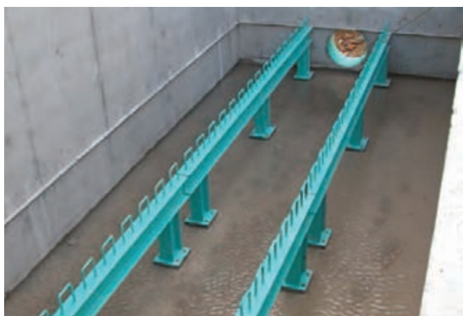
Alternative steel support structure.
