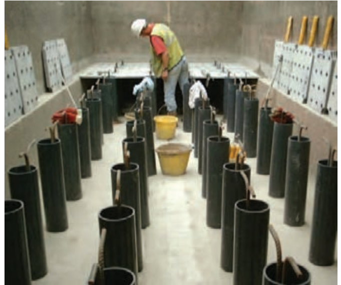
Plastic support tubes, cut to size and levelled.
